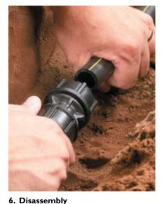
To disassemble the fitting simply loosen the nut using a wrench until 2 threads are showing. Pipe will be released and can simply be pulled out of the fitting.
