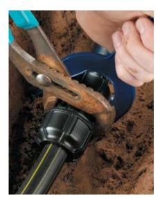
**4. Nut Tightening**The nut should be tightened by hand and then firmly with a wrench.
