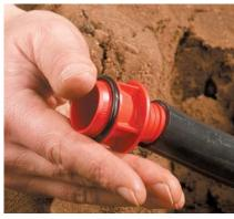
**4. Place Insert in Pipe**Remove the insert from the fitting and then place in end of pipe.
