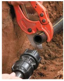
**I. Cut Pipe Square**Cut the pipe square. There is no need to prepare the pipe end.
